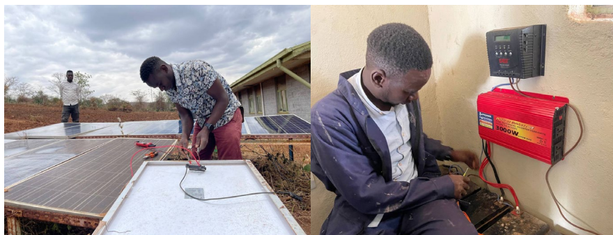
Repairing and upgrading Gotche Village Health Post Solar Power
